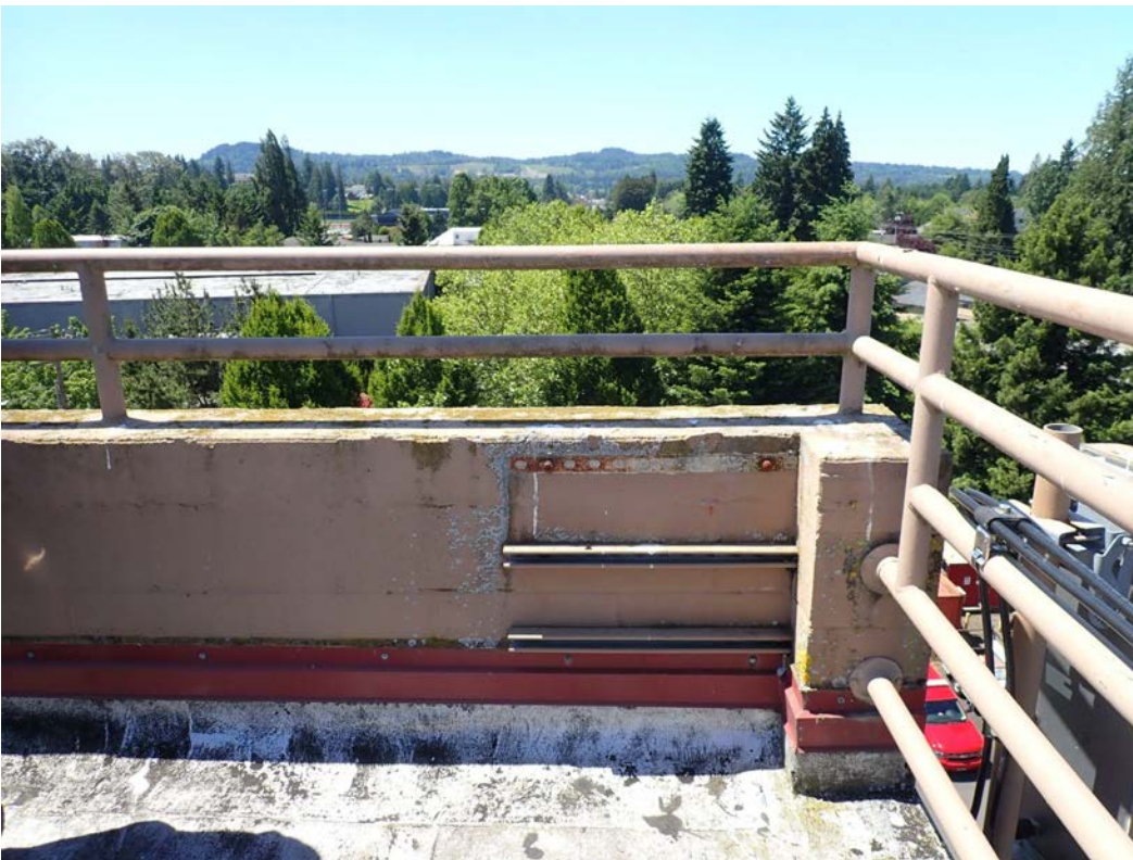
Image 10: Unistruts are mounted at each corner of the hose tower roof. A 5' antenna mast could easily be attached to these.
