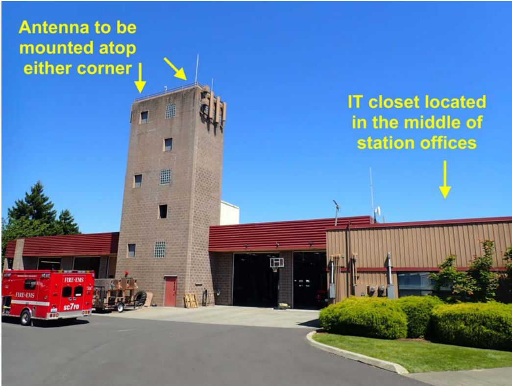
Image 1: Looking at the west face of Station 31.
