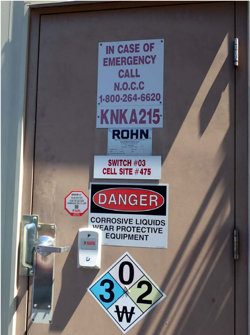
Image 4: Signs on the Verizon equipment room.
