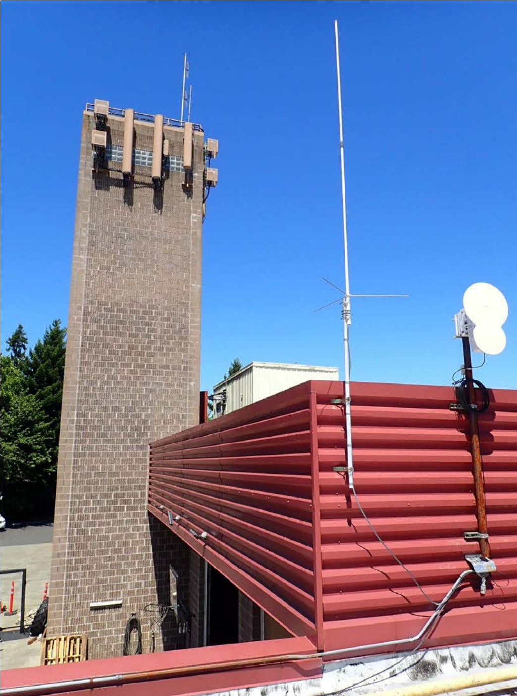
Image 12: Nearby Ubiquiti equipment and building penetration.
