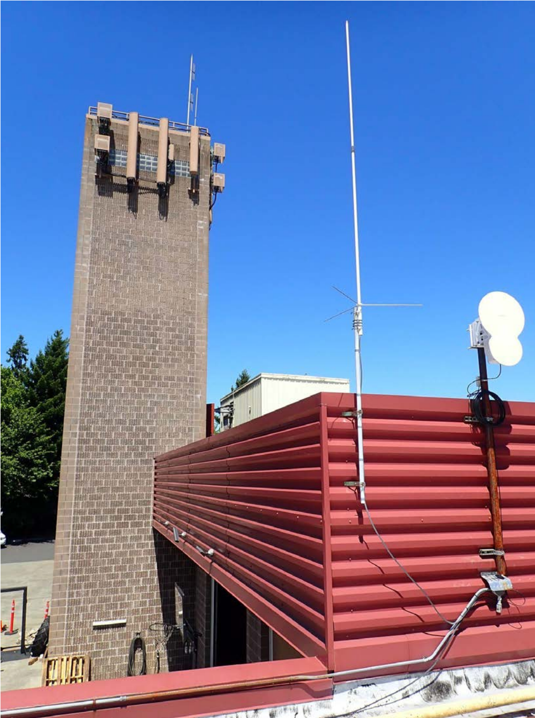
Image 12: Nearby Ubiquiti equipment and building penetration.
