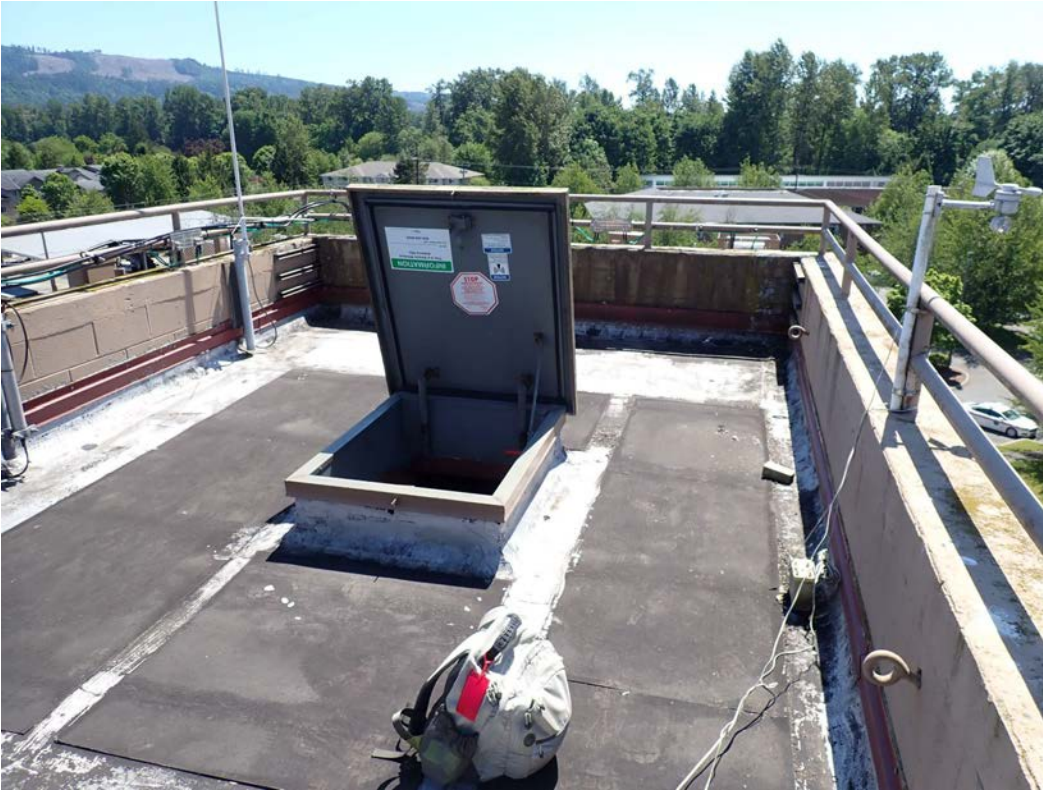
Image 9: View atop the hose tower.
