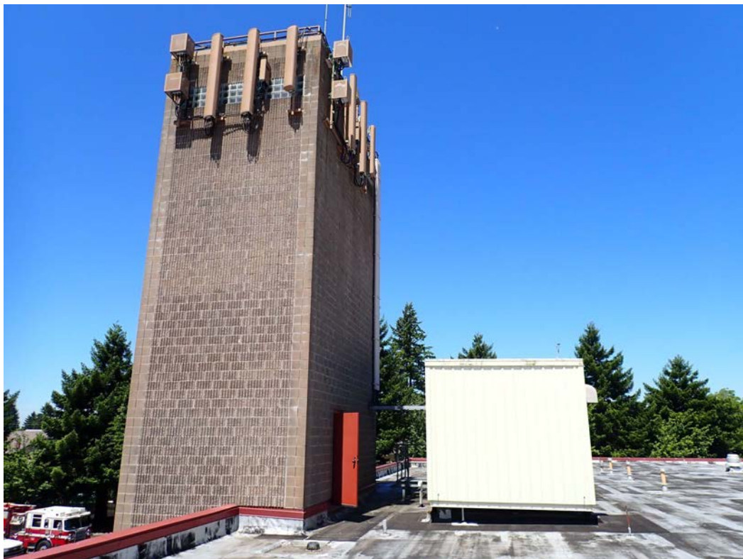
Image 2: Looking at the south face of the hose tower and Verizon equipment room on the station roof.
