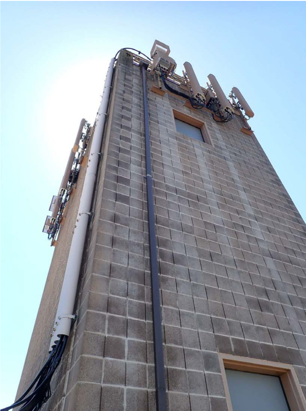
Image 3: Looking at the north face of the hose tower from the station roof.
