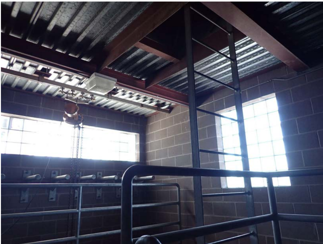
Image 6: The hose tower has stairs with a short ladder to the roof.
