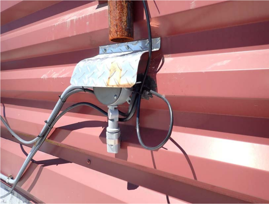
Image 13: Detailed view of the penetration.
